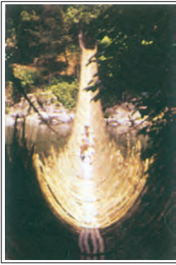
Figure 6.7 : Rope Bridge (Arunachal Pradesh)
