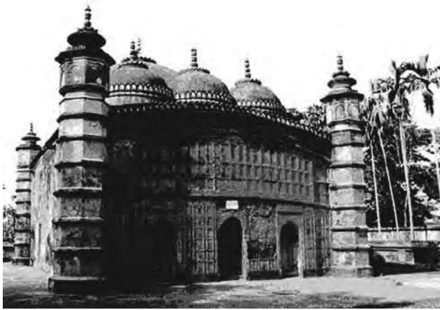
Fig. 6.10 Atiya mosque, Mymensingh district, Bangladesh, built with brick, 1609
